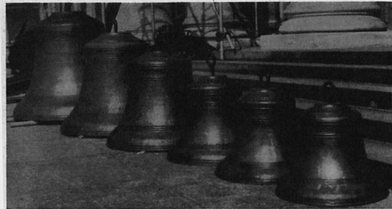
The Bells before installation in the Tower. Here all six bells lie at the foot of the steps leading up to the main entrance of the College. The notes and sizes of the bells are: G (2 cwt.), F (2½ cwt.), E flat (3¼ cwt.), B flat (7 cwt.), G (13 cwt.), E flat (25 cwt.). The four smaller bells are used for the Westminster Chime, the four larger ones for sounding 'Retreat.'
