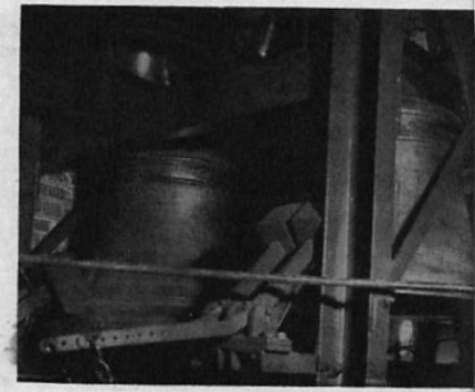
The larger bells, showing the arrangement of the hammers
